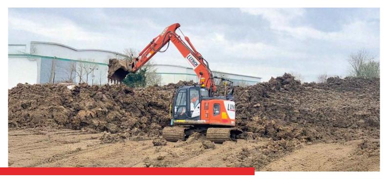
Lynch operates a modern and reliable fleet of bogmasters, specialised excavators designed for work on soft, marshy, or boggy terrain.
